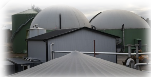
Overview of biogas plant in Vårgårda-Herrijunga Biogas AB in Vårgårda, Sweden
